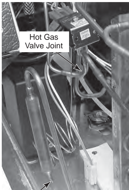
Drier Filter Capillary Tube
