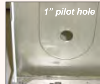
Marking center of pilot hole
