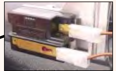
Bi-metallic Flame sensor closed
