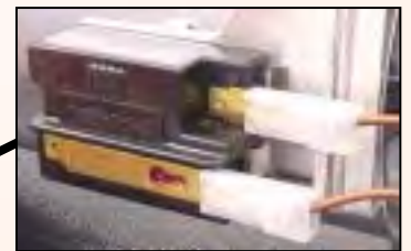
Bi-metallic Flame sensor open
